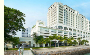
Eastern & Oriental Hotel Penang, Malaysia 6,000 m 2 Alum. Windows & Doors Completion 2012
