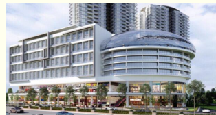
Sphere Damansara Plaza Kuala Lumpur, Malaysia Skylight, Alum. Windows & Doors
